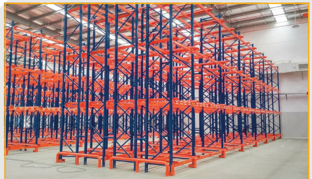
DOUBLE DEEP PALLET RACKING
