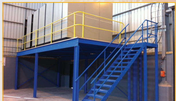
STEEL STRUCTURAL MEZZANINE
