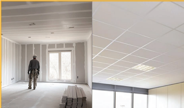
FIT OUT WORKS
