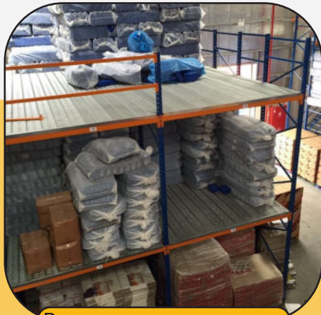
RACK SUPPORTED MEZZANINE FLOOR
